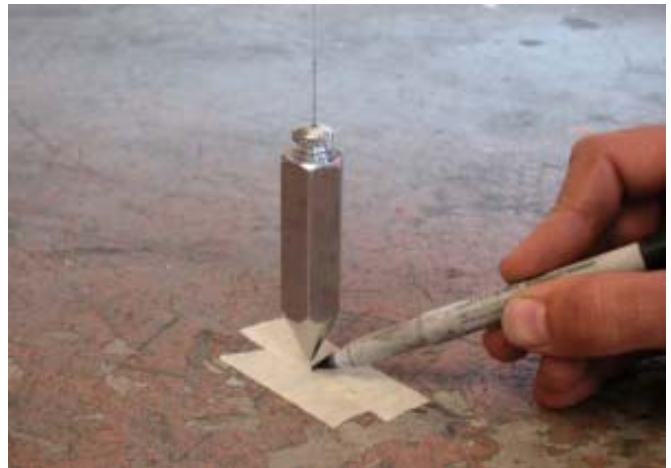
46. Wait for the plumb bob to stop swinging. Mark the position of each plumb bob by placing a small dot on the tape directly under the tip of the plumb bob.
