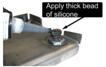
32. Place a large bead of silicone around the perimeter of the ½" holes drilled in Step 25.
