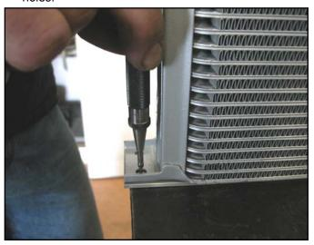
9. Drill out holes with 5/32" drill bit and de-burr.
