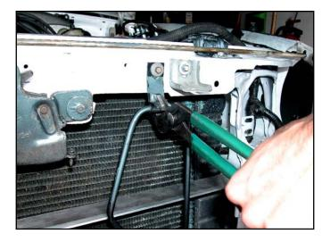
18. Center punch the marks for the top fittings on the upper L-bracket and using a 1-1/2" holesaw drill ONE of the holes for the top fittings on the cooler.
