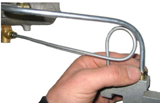
7. Tighten the ends of the brake hard lines to 12-16 ft-lbs at the master cylinder and the proportioning valve.
