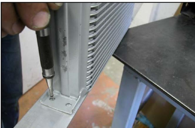
21. Drill out holes with 5/32" drill bit and de-burr the holes.
