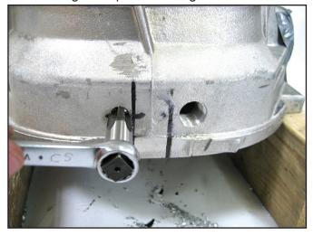
91. Periodically unthread the tap and clean the threads of any metal chips. After cleaning, apply more lubricant to the tap.
